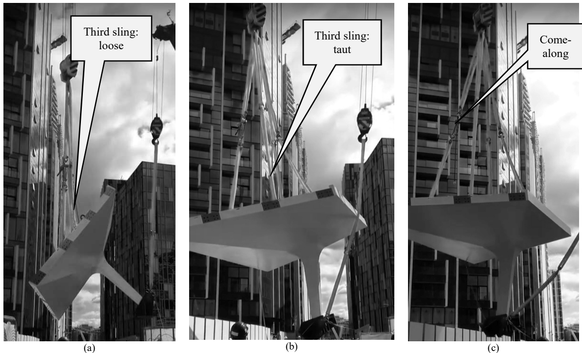
Figure 16: Phases of the rotation operation. (a) Beginning of the rotation operation. (b) Activation of the third top sling preventing additional tilting of the module. (c) Last phase of the rotation operation.
