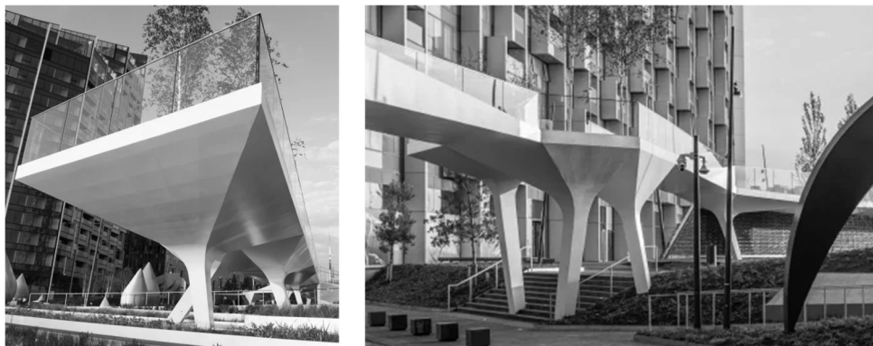
Figure 1: Footbridge in London, UK. Source: [1]
